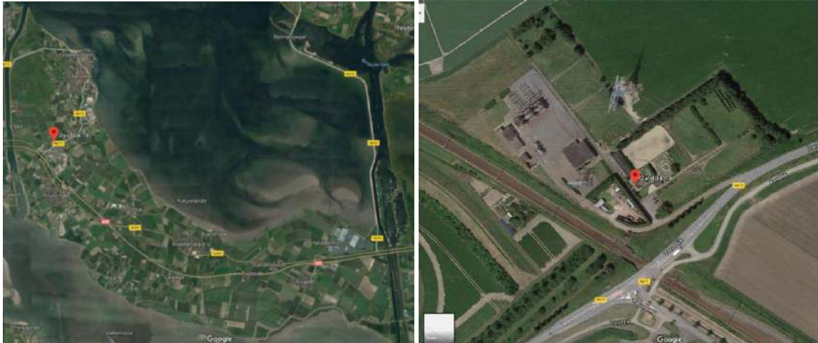
Figure 5.4 Location and aerial photo of high-voltage supply station
