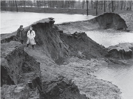
Figure 1 Pictures of the 1953 flooding in the Netherlands (top) and Belgium (bottom). This flood was caused by a levee break due to high tidal waves.
