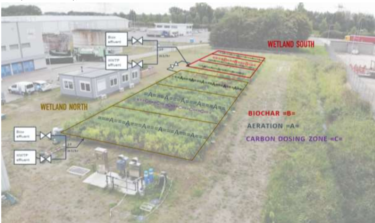
Figure 4: Overview of two Constructed wetland pilots at DeCo.
