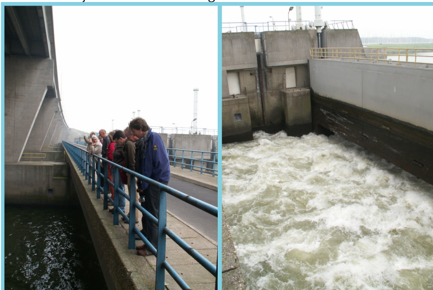
Figure 5.1 Visit to the Volkerak locks and sluices. By coincidence the committee could witness a test discharge at maximum capacity at the sluices.
