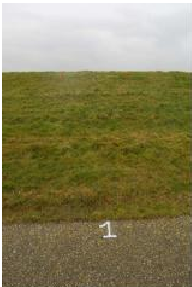
Test strip 1, overview
