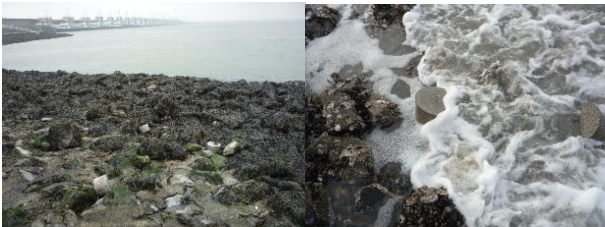
Figure 8. All that remains of the field experiment in some locations were the concrete blocks strewn in the kreukelberm. Here the concrete blocks at Neeltje Jans Buiten.
