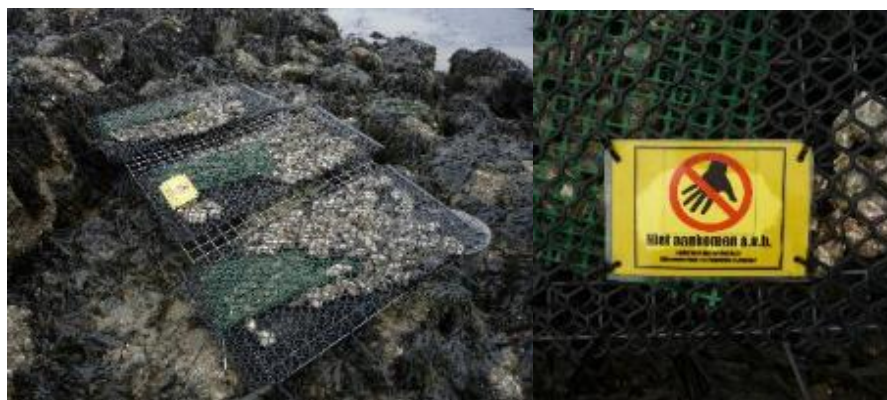
Figure 6. Oyster sacks (with small oyster bag inside) attached to the steel sheet, weighted by concrete blocks and placed on the kreukelberm (left) and signage intended to dissuade potential oyster thieves placed with each set of oyster sacks (right).
