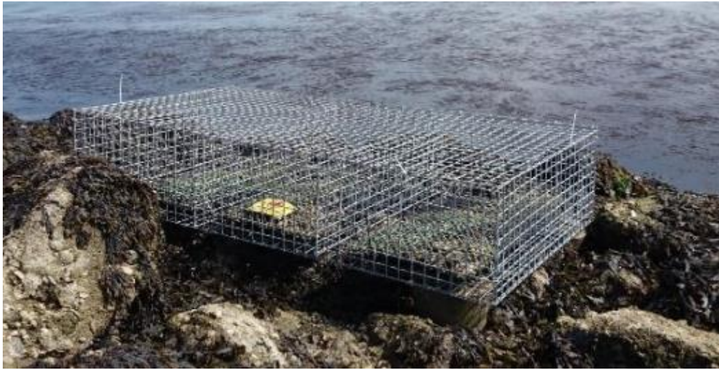
Figure 7. Steel gabion with oyster sacks in locations where increased security for the oysters was necessary.
