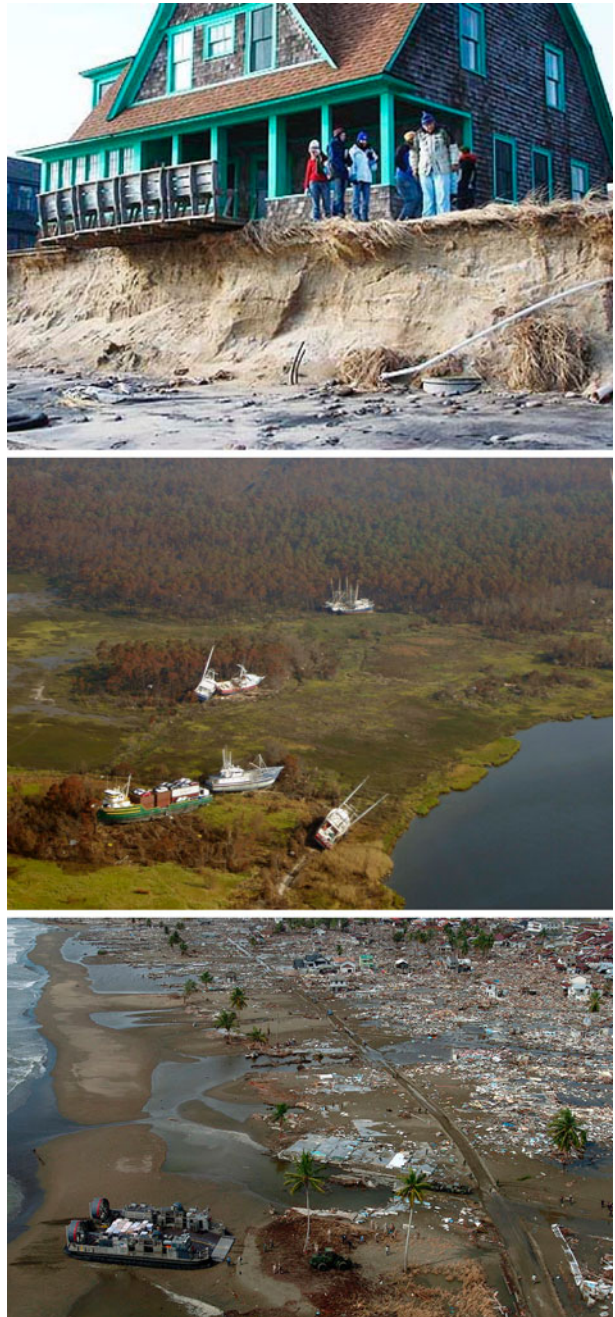
Fig. 1 The risks of the living along the shore: a Coastal erosion in Rhode Island, USA has severely compromised a home ( http://celes.uri.edu/news/nBoothroyd.aspx , URI College of the Environmental and Life Sciences). b Boats pushed ashore in the storm surge of hurricane Katrina, September 2005 (NOAA). c A U.S. Navy hovercraft brings aid to Meulaboh, Sumatra, Indonesia on Jan. 10, 2005, just days after it was decimated by the 2004 Indian Ocean Tsunami (U.S. Navy)
