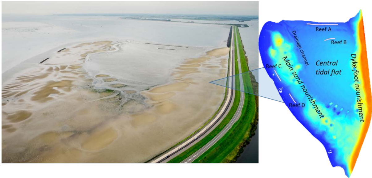
Figure 2. The sand nourishment at the Oesterdam and placement of the constructed oyster reefs (Photo by Edwin Parea, Rijkswaterstaat).
