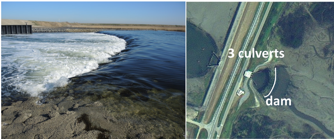
Figure 3 Left: Outflow of saltwater during ebb from the Rammegors (right side of photo) into the Oosterschelde through the three culverts in the Krabbenkreekdam (left side of photo). Photo: Tom Ysebaert. Right: Position of the dam in the Rammegors area and the three culverts in the inlet.
