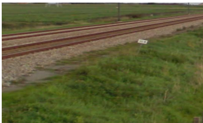
Figure 58 Grass revetment on location 2 (Googlemaps, 2018)
