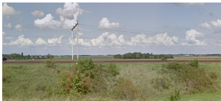
Figure 59 Grass and trees on location 3 slope (googlemaps, 2018)
