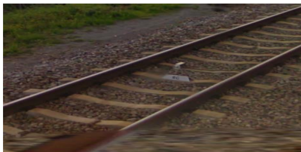
Figure 13 Sleepers in existing railway structure (google maps, 2018)
