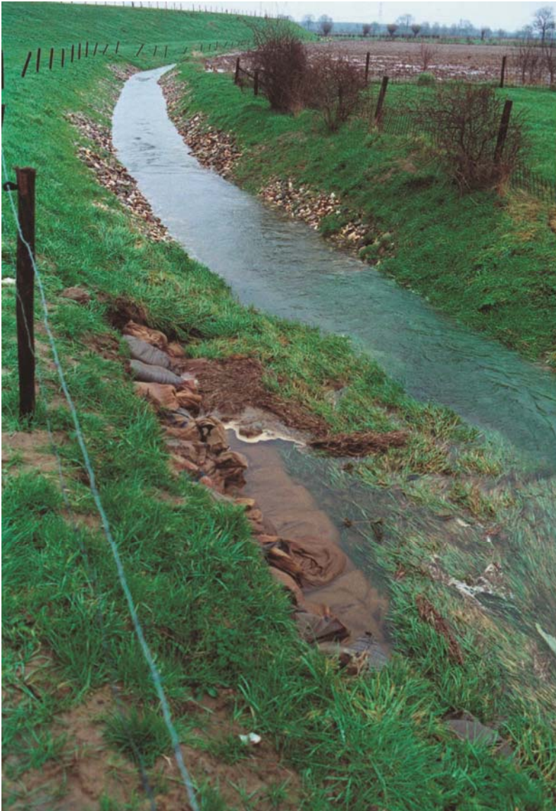
2.15b: Verzakte slootberm. [RWS-DWW 905_11]
