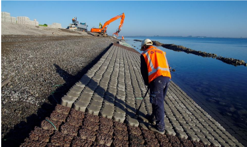
Fig. 2. The placement of the revetment at Sint-Annaland during spring 2015.
