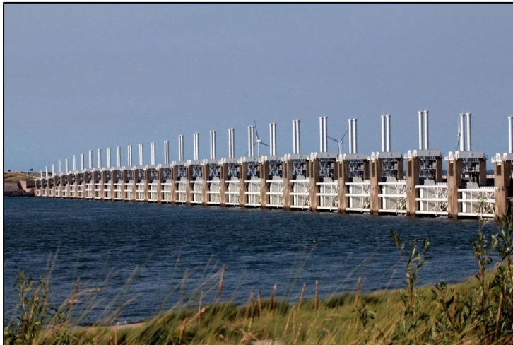
FIGURE 5: THE EASTERN SCHELDT STORM SURGE BARRIER (FLETCHER, 2012)
