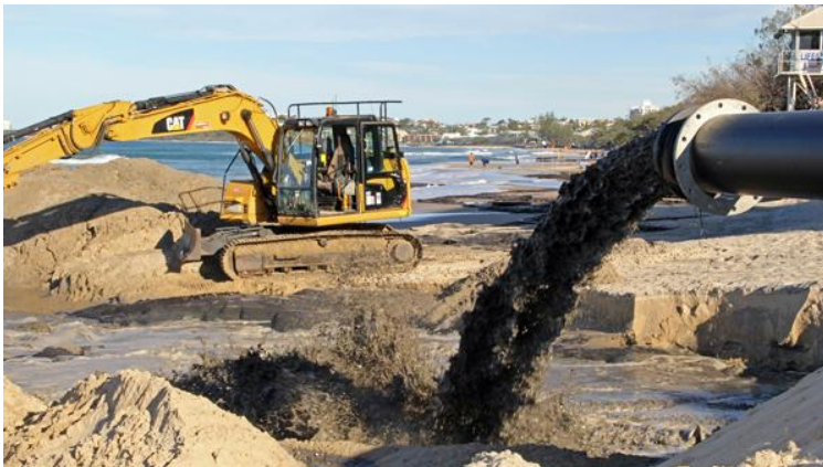
Figure 2.8 – How to realize a sand nourishment
