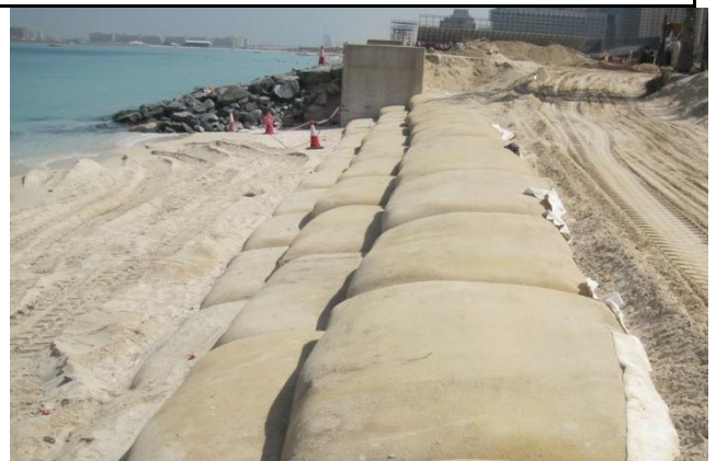
Figure 2.24 – Examples of geocontainers for coastal protection (www.ecobarrier.ae)
