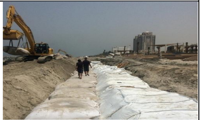
Figure 2.26 – Example of barriers of bags filled with sand (www.ecobarrier.ae)
