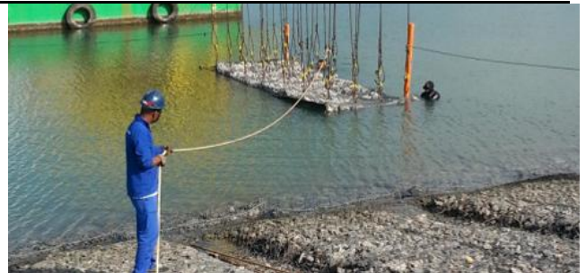
Figure 2.22 – Example of gabions filled with stones (www.maccaferri.com)
