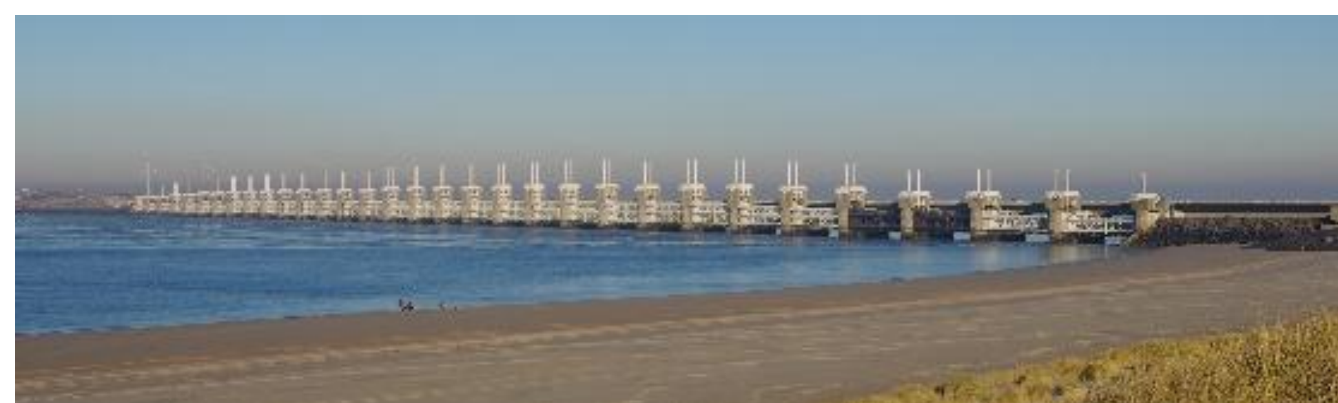
Figure 2: The Eastern Scheldt storm surge barrier. [Tjark van Heuvel]
