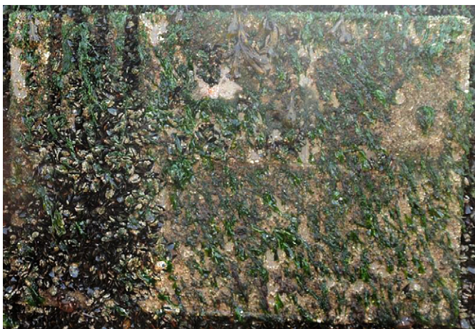
Fig. 3. Photograph of the slab (Fig. 2) after 17 months at a low dynamic position low in the intertidal area. High densities of mussels ( Mytilus edulis ) were found at the groove structures and low density of mussels were found at the hole structure, whereas mussels were absent at the other sections of the slab.
